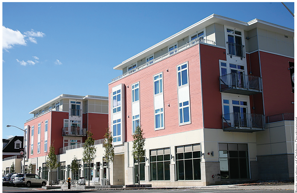
Reading's smart growth district zoning attracted projects such as Oaktree Development's 30 Haven, which includes 53 apartments and 22,000 square feet of retail space steps from an MBTA commuter rail station.
