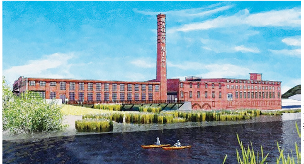
State and federal historic tax credits generated $13.5 million in equity toward the first phase of the Eagle Mill redevelopment in Lee which began construction this spring. Rees-Larkin Development and Berkshire Housing Development Corp. are creating 56 affordable apartments in the complex, which operated as a paper mill from 1808 to 2008.
